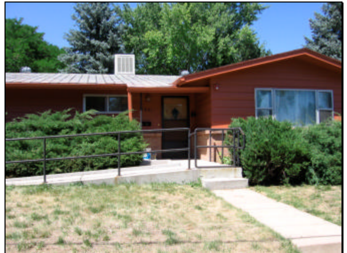
View of the front entry.
